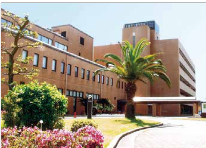
Fig. 1 Nagoya Municipal Industrial Research Institute
