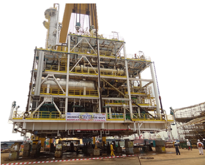
Example of a typical FPSO process module, which is inserted on top of the FPSO.
